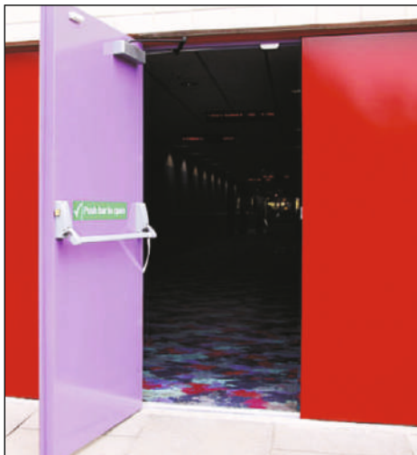
Metal Fire Rated Door
